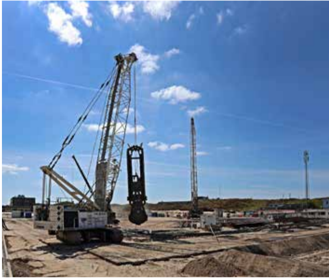
Works on diaphragm walls
