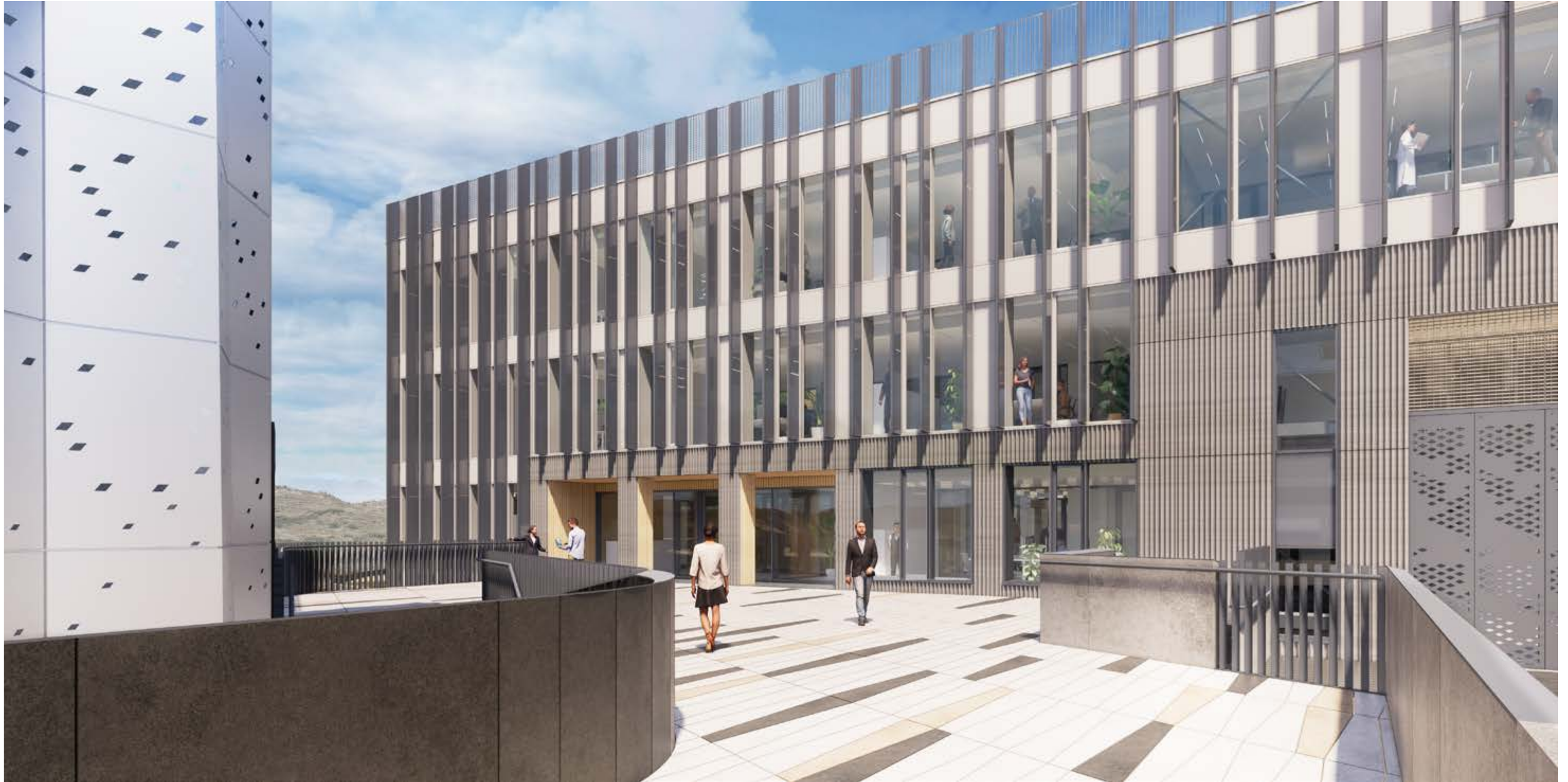
Entrance of the support building.
