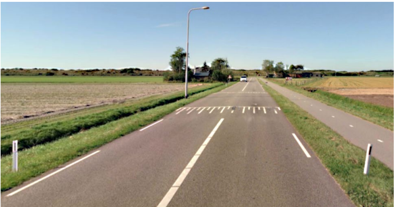
Figure 75 N503 at the Belkmerweg (top) and between the N502 and Bosweg (bottom, Source: globespotter)
